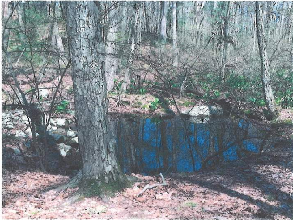
Photo 23. Stone catch basin at Pine Spring. Photo by Ann Clifford, 2019.
