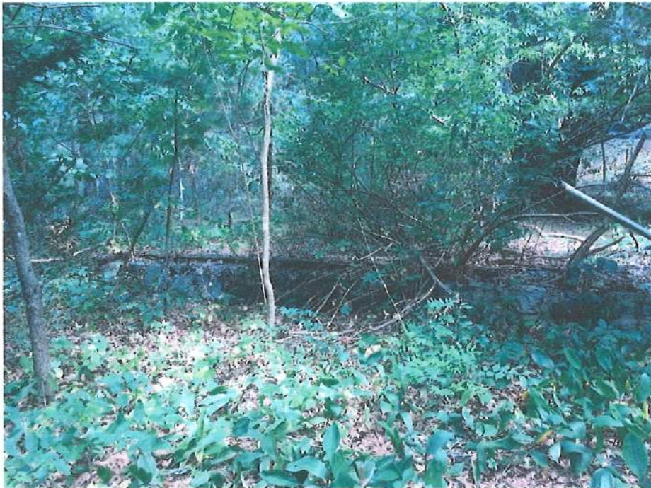
Photo 25. Storer outbuilding foundations. Photo by Ann Clifford, 2019.
