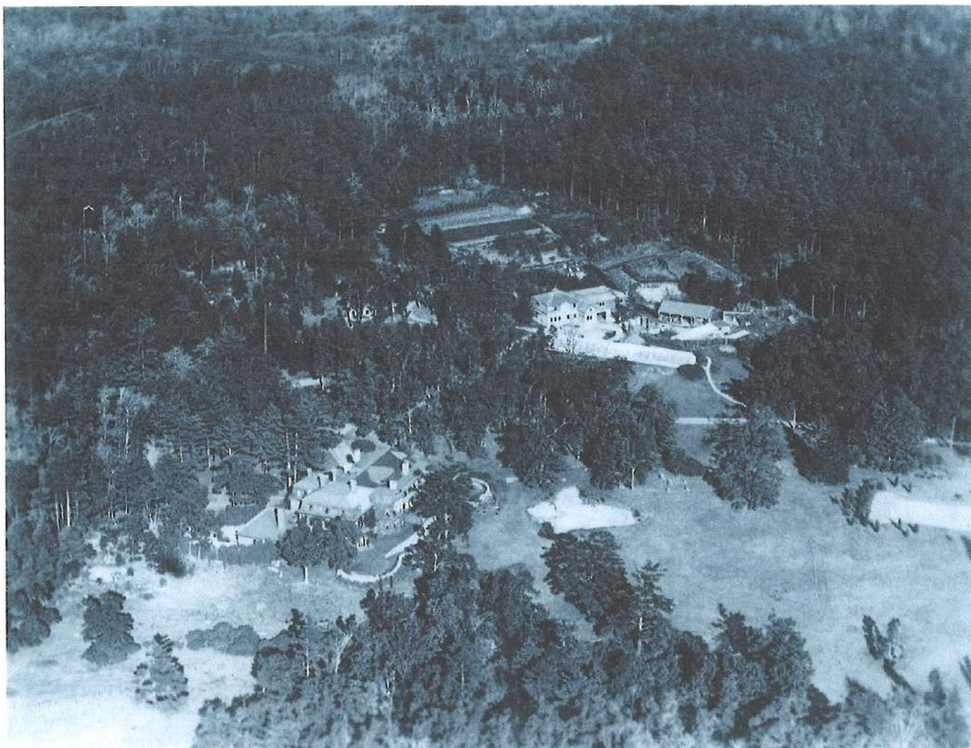
Figure 1. Aerial View of the Robert Treat and Lydia Lyman Paine Family House (H.H. Richardson, 1886 and Gridley J.F. Bryant, 1866) and its site (Frederick Law Olmsted, 1886) known as Stonehurst. Ernest Bowditch sited the outbuildings and designed the greenhouse. Photo, November 1924. Stonehurst Archives.
