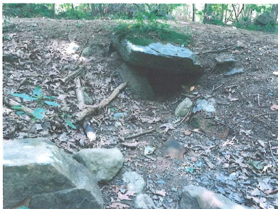
Photo 22. Representative stone culvert that seasonally channels spring water under a cartpath to an old orchard. Photo by Ann Clifford, 2019.
