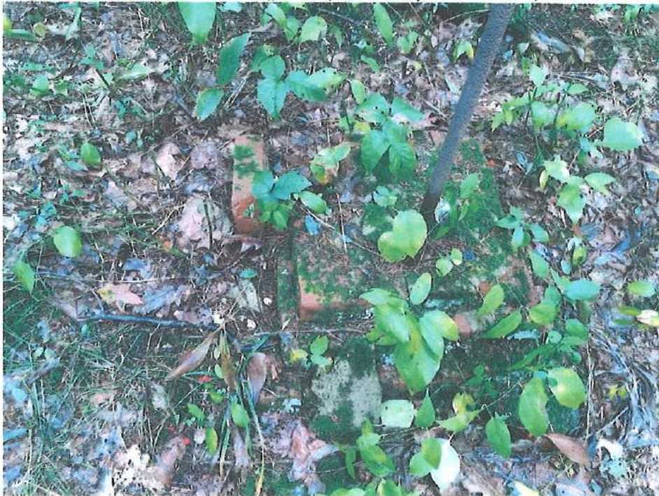
Photo 14. Windmill foundation 1. One of eight supports arranged in an octagon. (See Figure 13). Photo by Ann Clifford, 2018.
