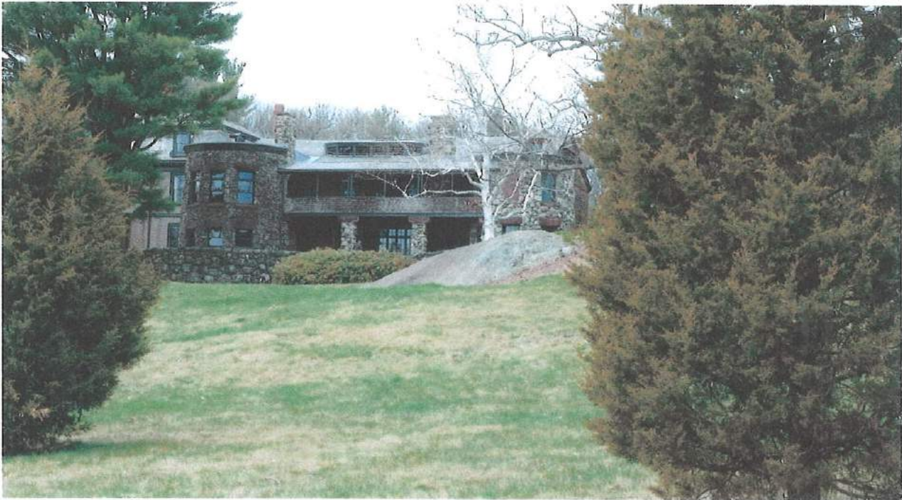
Photo 5. Grounds: former site of 1866 house and outbuildings. The 1866 Second Empire house is shown here in its new location to the west of the stone Richardson-designed addition. Photo by Thomas P. Lang, 2007.
