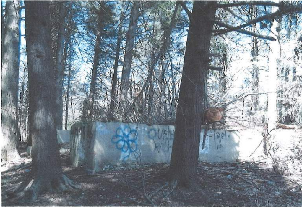
Photo 17. Modern cement foundation built atop historic foundations for cold storage for apples and pears. Photo by Ann Clifford, 2016.
